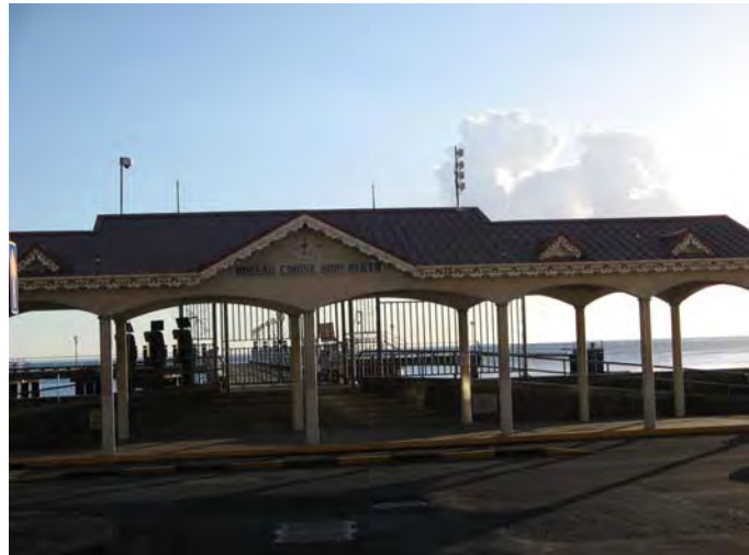
Ferry Terminal: Roseau
